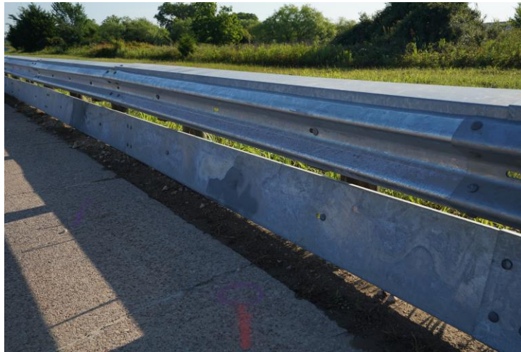
Figure 1.1. Wood Post MGS with Motorcycle Rail Elements. (2)
